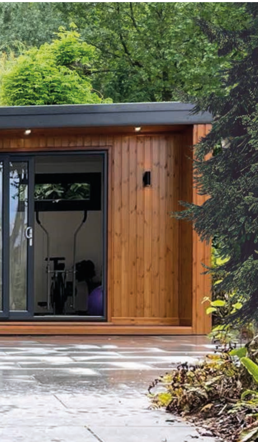
22' x 14' Haven with uPVC windows, single sliding door and 10' integral open sided area
