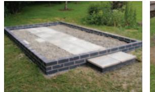
Your base will affect the long term strength and stability of your greenhouse, so it is worth investing at this stage. It is vital that your greenhouse is anchored down to the base. With most models we supply L-shaped brackets and screws & rawl plugs for this purpose.
