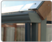
Guttering and downpipes
