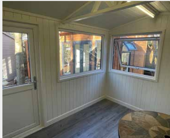
10' X 8' Apex garden studio. thermowood cladding, UPVC doors & windows slate grey, satin handles & levers & grey hinges, half length single door, half length opening window (1000 x 1200) & half length fixed window (1000 x 1400), double glazed, MDF (V grooved) painted lining (white) with breathable membrane (moisture barrier) & Celotex insulation, painted finish in elephant grey, EPDM rubber roof, laminate floor midnight grey.
